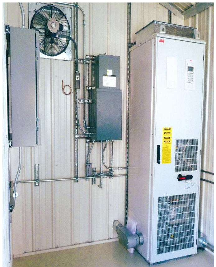
Compressor 300 HP Low Harmonic VFD
