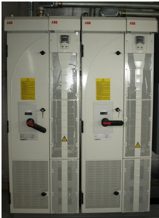
ABB Snowmaking 300 HP Low Harmonic VFDs
